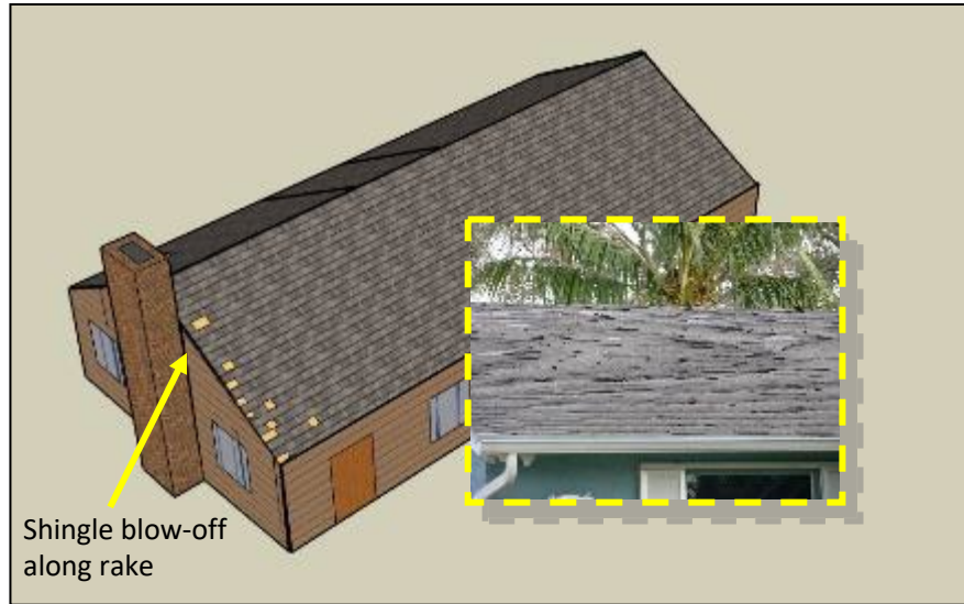
Category 1: Minor loss to roof covering
